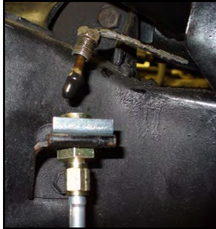
Figure 1: Vinyl cap installed onto hardline
